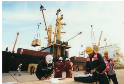
Generation project Campana's port
